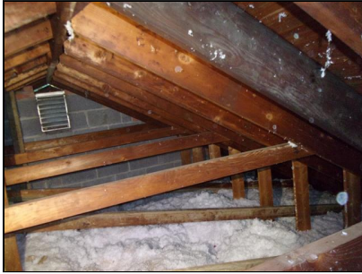
1.7 Item 1(Picture) Attic insulation
