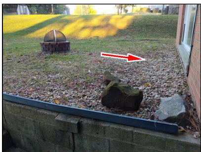
2.4 Item 5(Picture) Ground slopes toward foundation
