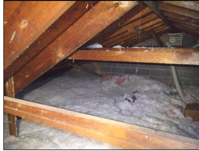
1.7 Item 2(Picture) Attic insulation
