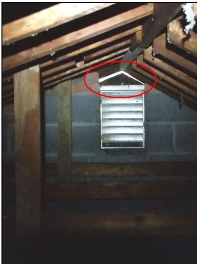
1.5 Item 1(Picture) Gap over passive vent
