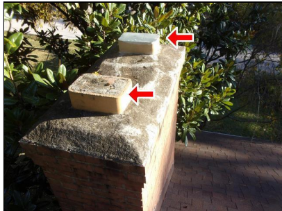
10.6 Item 2(Picture) Flue pipes sealed
